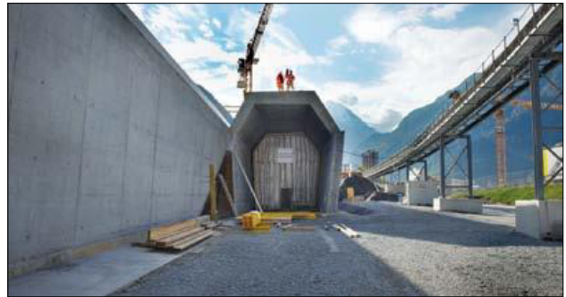
Northern portal structure of the 57-km-long railway tunnel near Erstfeld, Switzerland.
