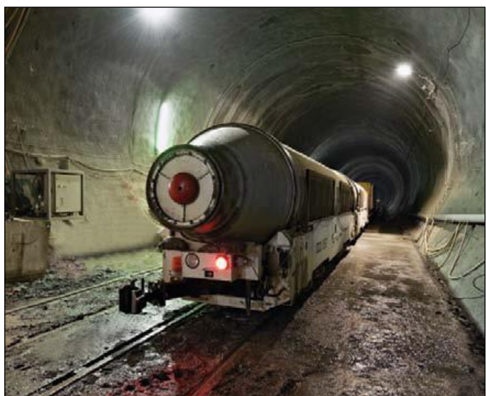
Concrete transport train in the tunnel.
