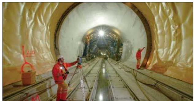
Checking the inner concrete formwork using a Trimble S8 Total Station.
