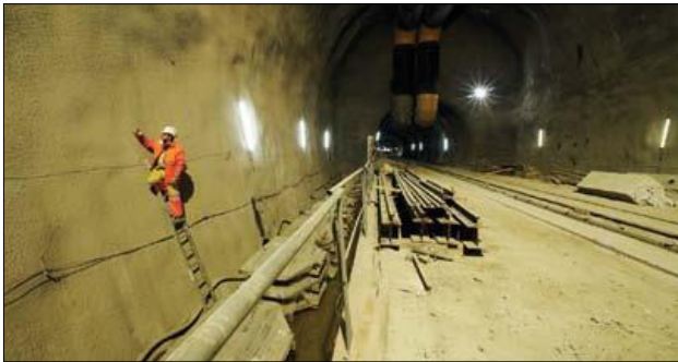
Mounting bi-reflex targets for convergence monitoring.
